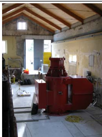
Synchrongenerator 2.4 MVA
